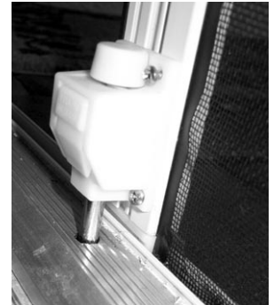
Double door stop pins(come as a pair). The pin on the right has been mounted with a hole directly in the threshold- the keeper plate was not used.
