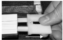
Step 4) Loosen the set screw on the Dreamscreen handle on the side of the door you are installing the stop pins and slide the handle out.
