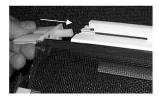
Once the Dreamscreen doors have been installed, mounted the keepers (included in the stop pin parts bag) to the top and bottom of the door frame.
